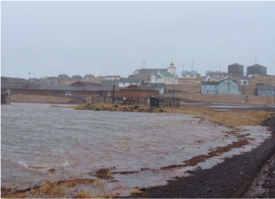
The Pond filled with sea water from the storm surge reaching the Sandy Lane Sewer Lift Station and Ball Field.
