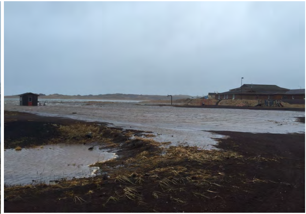
The Pond filled with sea water from the storm surge going onto the Ball Field.
