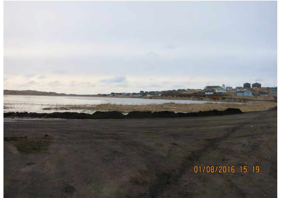
The Pond filled with sea water from the storm surge reaching Bartlett Boulevard and Reef Road intersection and a dirt berm constructed to prevent further flooding of the roads.
