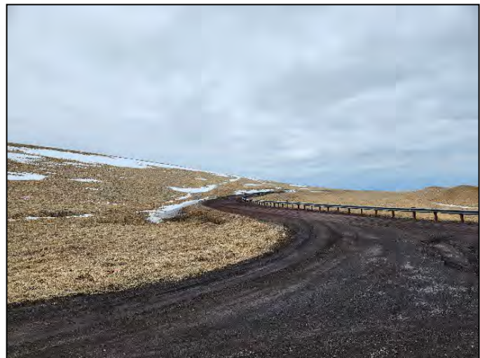
Policy review included determining location of and replacement need for Proven Safety Countermeasures, including guardrails.
