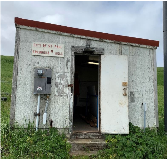
North Well House
