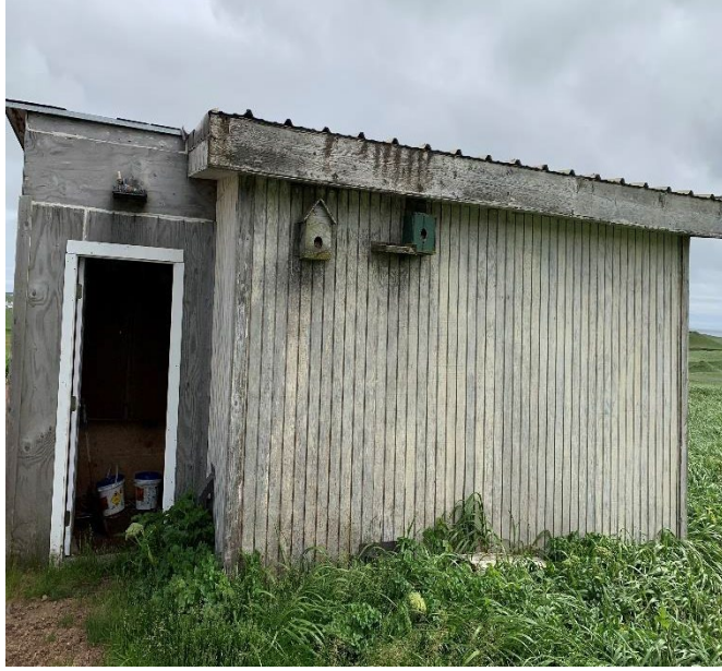
Water Treatment Plant
