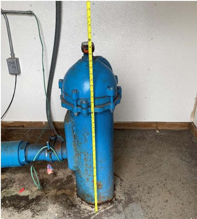
Photo 40: Well casing measured at 25 inches above floor.
