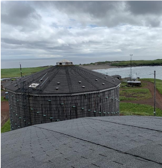
Photo 57: Top of WST 2 in good condition.
