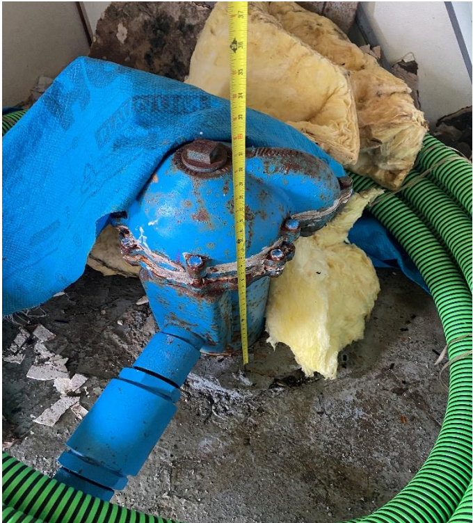
Photo 36: Well casing measured at 20 inches above floor.
