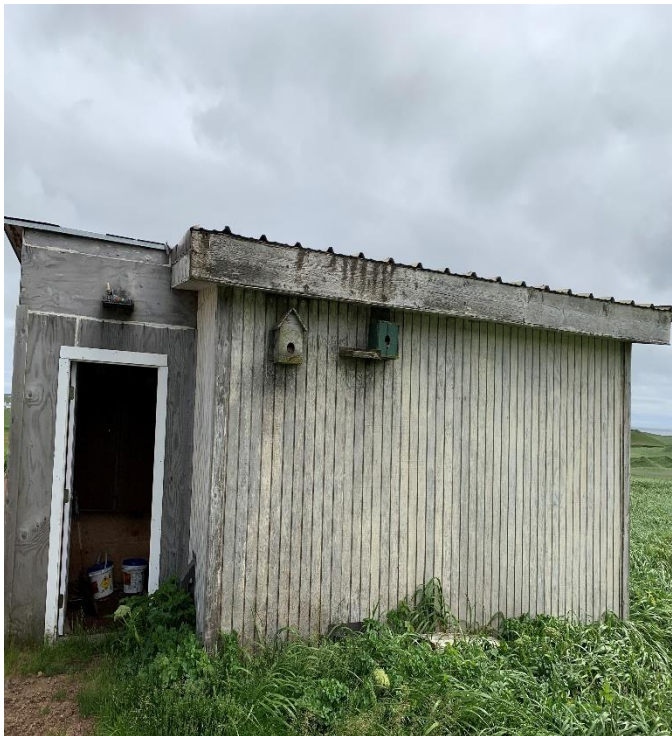
Photo 44: Exterior of WTP in good condition.
