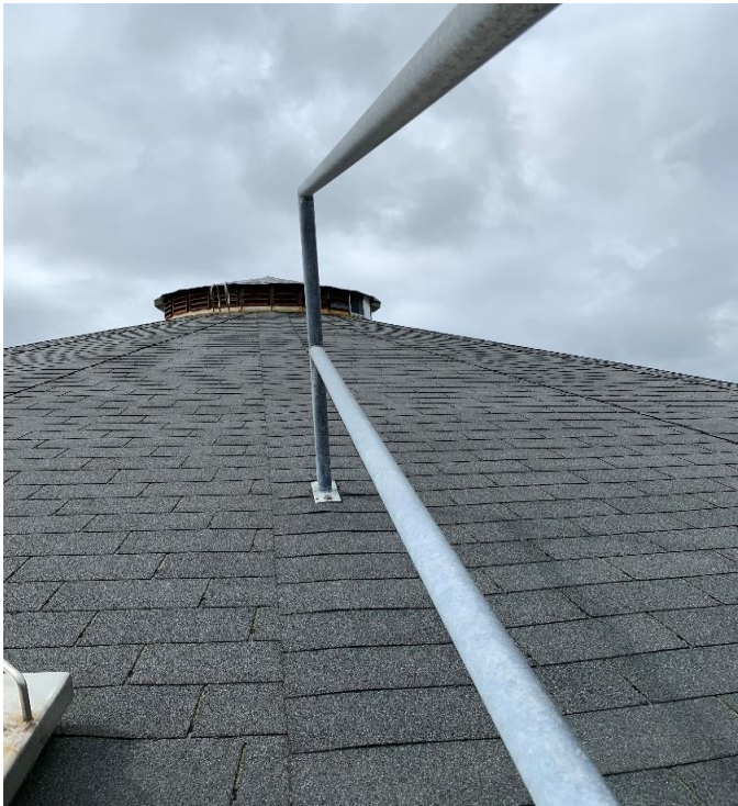
Photo 50: Top of WST 1 in good condition.
