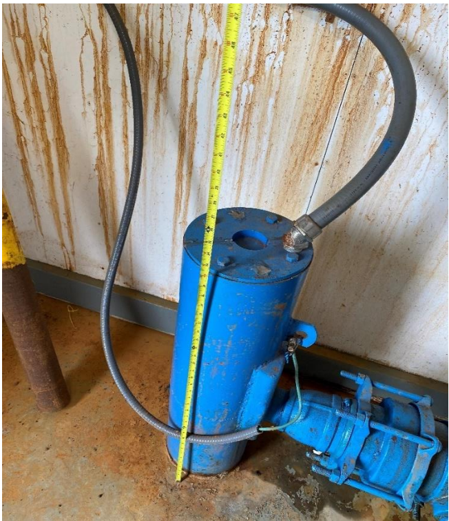
Photo 28: Well casing extending 32.5 inches above floor.
