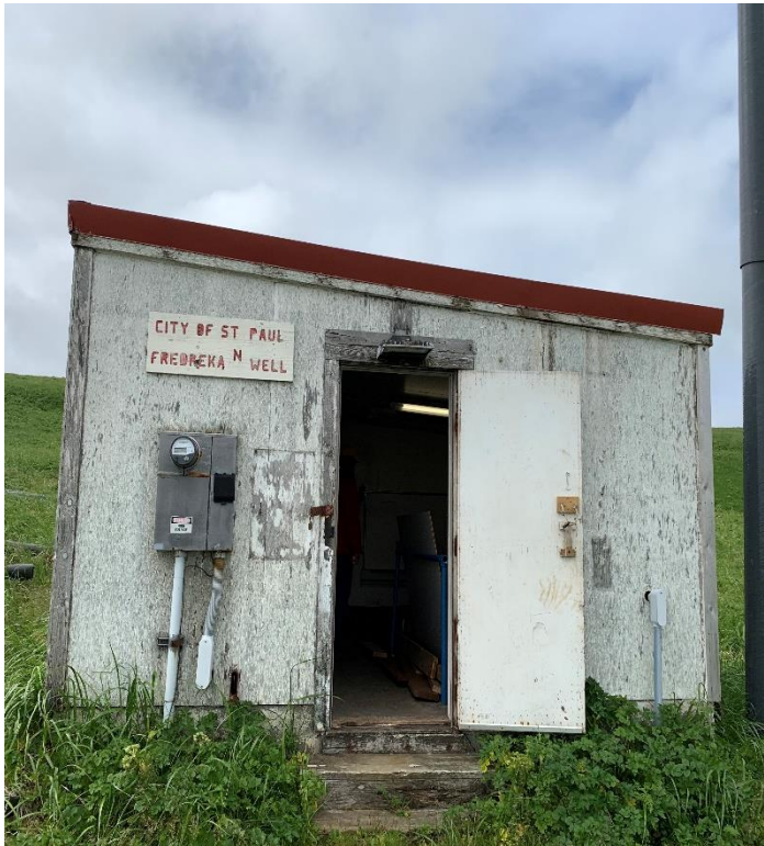
Photo 8: North well house building in good condition.
