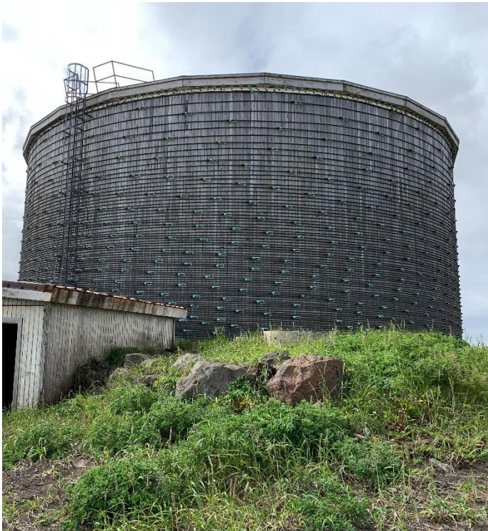
Photo 59: Exterior of WST 1 in good condition.
