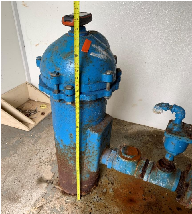
Photo 31: Well casing measured at 30.5 inches above floor.
