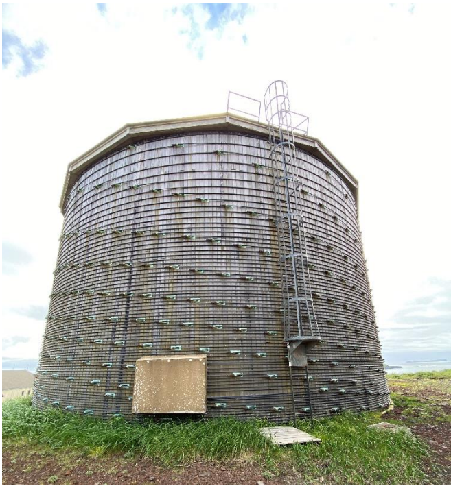
Photo 58: Exterior of WST 2 in good condition.
