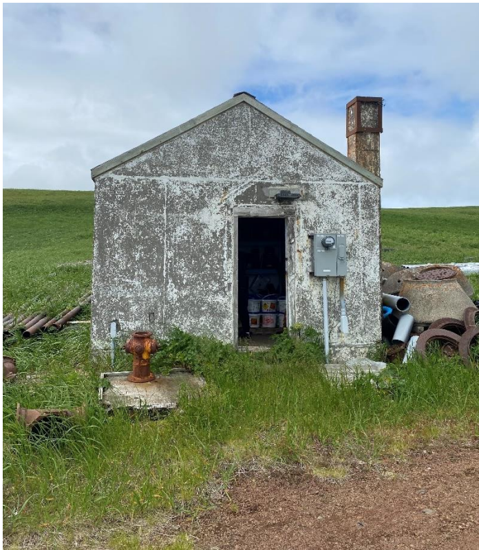
Photo 1: Well house building in good condition.
