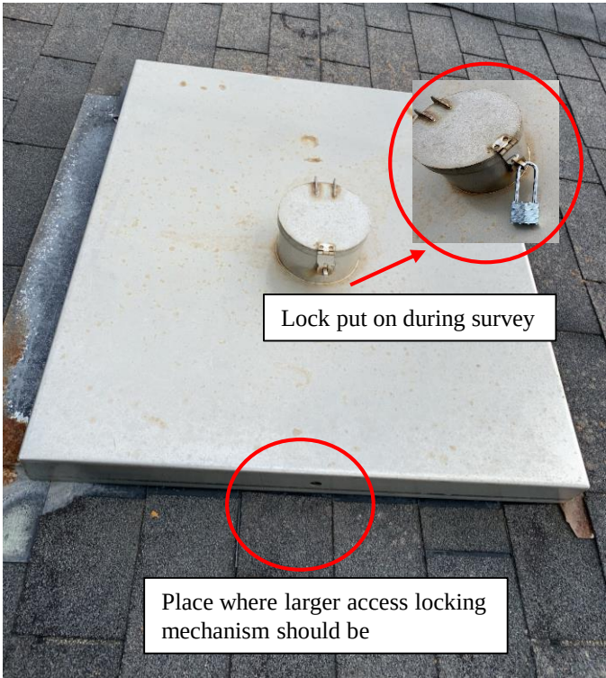
Photo 55: Smaller access hatch on WST 2 locked.
