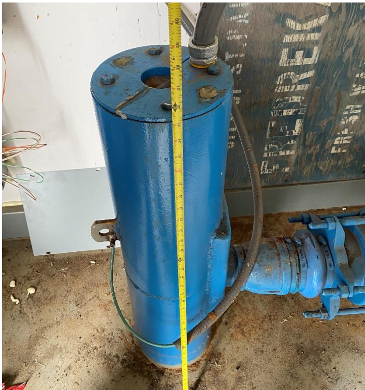
Photo 20: Well casing extending 35 inches above floor.
