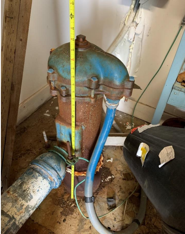
Photo 2: South well casing 29 inches above floor.
