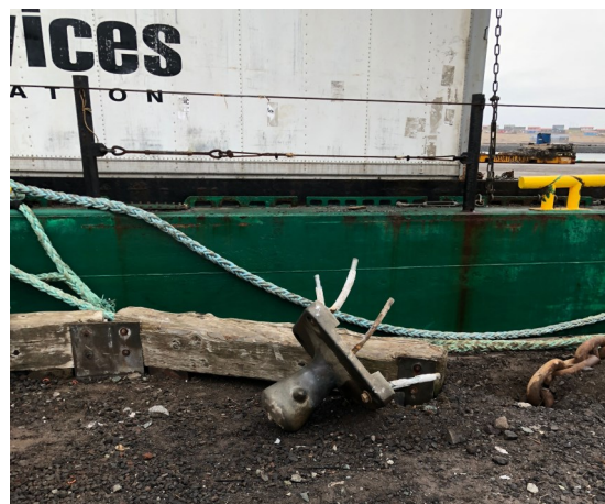
Figure 11: Mooring bollard ripped out by barge at City South Dock
