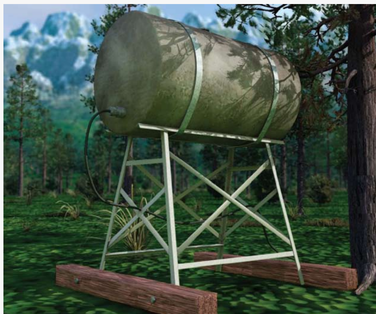
Secured Elevated Oil Tank
