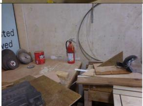
Extinguishers should be mounted on brackets or in wall cabinets with the carrying handle placed 3-1/2 to 5 feet above the floor. NFPA 10 6.3.1.1
