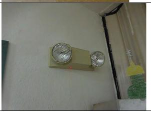
Electrical wires must be completely enclosed to prevent an employee from accidental electrocution. 1910.305(b)(2)
