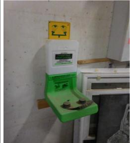
Eye wash stations must be run on a weekly basis and need to have their protective covers on. ANSI Z 358.1-2014
