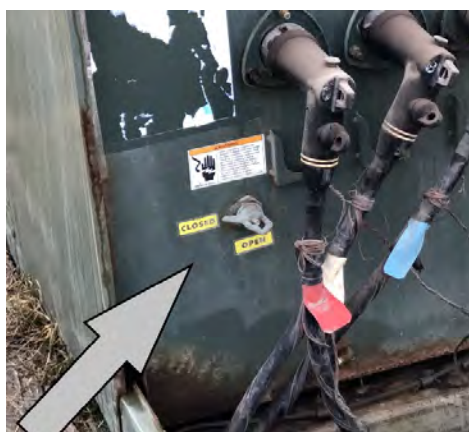
PIC 1. R7 Switchgear- Showing the switch in the closed (energized) state.
