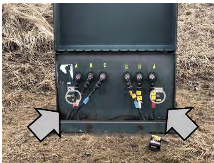
PIC 2. R7 Switchgear- Showing the location of switches per covered side.
