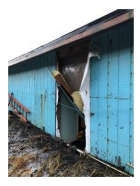
The team then entered the building to assess that interior damage. There was evidence of water flooding the office through the damaged wall as there were debris and dirt/mud throughout the building interior (see photos below).
