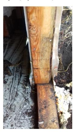
There is evidence that more of the wall is pushed in on both sides of the damaged area, which is indicated by the cracks in the sheetrock in the bathroom (*see photos*).
